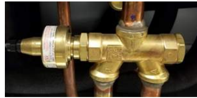
Figure 2: Modulating Hot Gas Reheat Valve
