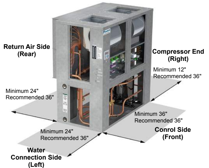
Figure 18: Service Clearances
