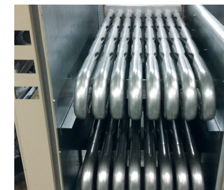
Gas Furnace Tubes
