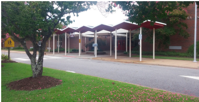
Low roof and ceiling clearances necessitated rooftop units to replace exterior wall-mounted unit ventilators.
