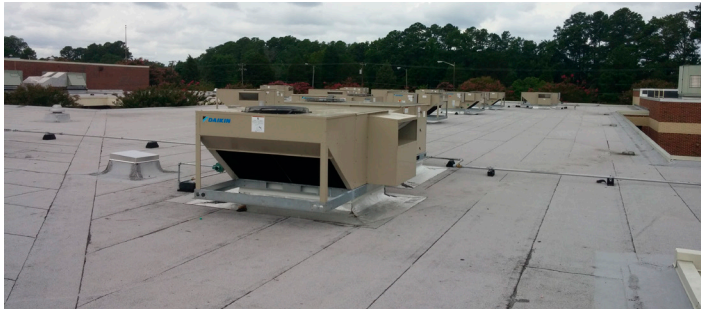
Lightweight Rebel units and versatile installation required minimal structural considerations to the facility.
